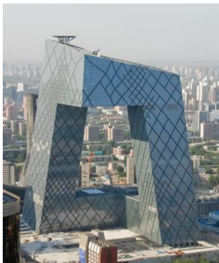
Figure 2.06 – The CCTV Headquarters designed by Rem Koolhaas with the structural counselling of the Advanced Geometry Unit (source: https://aedesign.files.wordpress.com )
