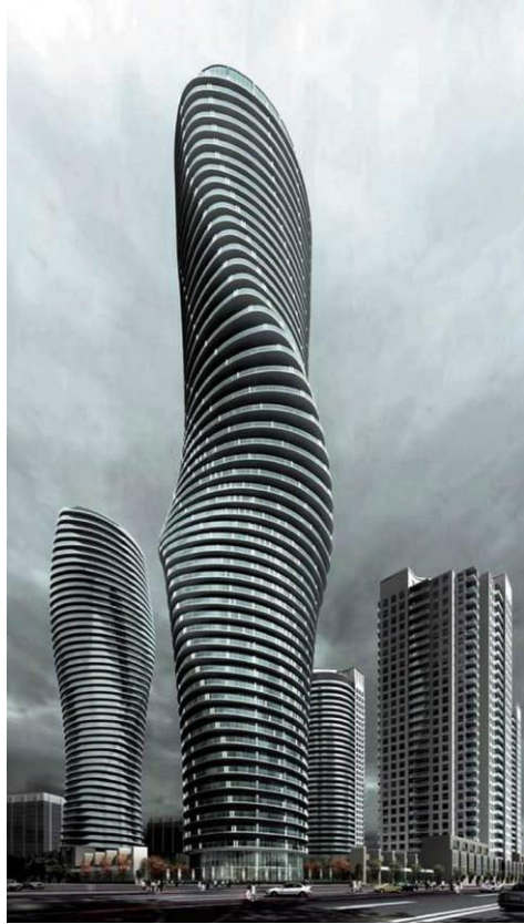
Figure 5.01 – The Absolute World Towers, designed by MAD Architects (source: http://www.e-architect.co.uk/ ).
