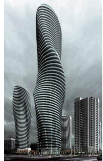
Figure 4 – The Absolute World Towers, designed by MAD Architects (source: http://www.e-architect.co.uk/ ).
