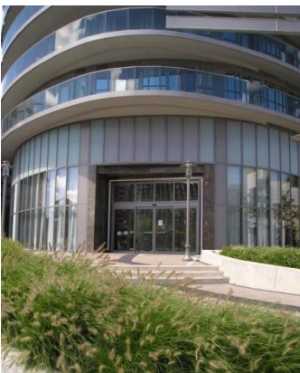
Figure 9.09 – Curved curtain wall in the ground floor of the AWTs (source: www.randyselzer.com/ )
