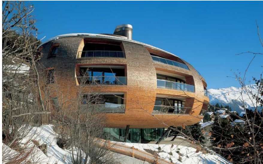
Figure 2.05 – The Chesa Futura apartment building designed by Foster & Partners with the support of the Specialist Modelling Group (source: http://www.fosterandpartners.com/ )
