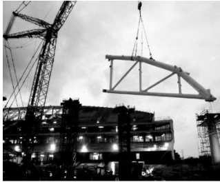
Figure 4.05 – Erection of the pre-fabricated steel work (source: Shepherd et. al., 2011).
