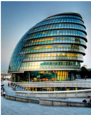
Figure 2.03 – Designed by Foster & Partners, the London City Hall's round and slightly tilted form was obtained through an optimization process: the surface in contact with direct sunlight was minimized, resulting in reduced solar gains through the building's skin. (source: http://www.theneweconomy.com/ )
